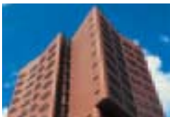
Officer's quarters of the Royal Marines of the Netherlands, Den Helder Van Herk & de Kleijn Architekten BV, Amsterdam Ridder BV, Hoorn TECU® Classic
