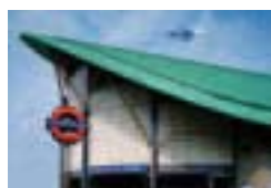
Underground station Hounslow West, London, GB Michael Watkins (Partner), London, (Acanthus, Lawrence and Wrightson Architects) Broderick Structures Ltd., Woking TECU® Patina
