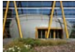
Administrative building of WeberHaus, Rheinau/Linx, D Dipl.-Ing. Günter Hermann, Stuttgart Wittenauer GmbH, Sasbach TECU® Zinn
