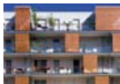
Residential Building "Le Galilée", Rennes, F Chouzenoux et Associés, Rennes SABM, Guichen TECU® Net Classic
