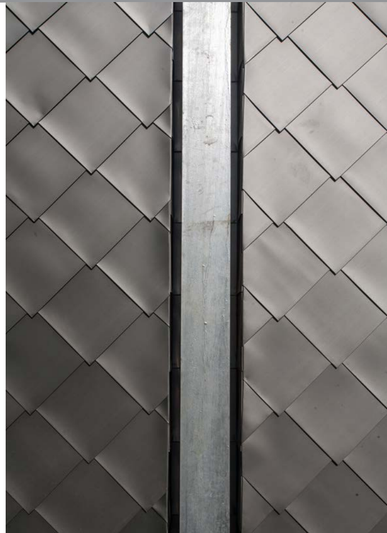
'A very honest, natural coloured material' NedZink NOVA shingles trim the dolphins. Photo © Baca Architects
