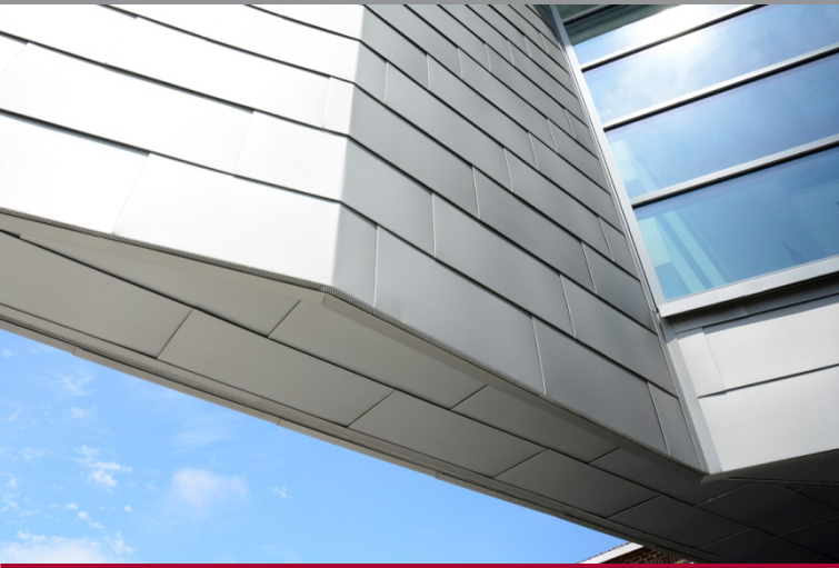
Non-centered shingle set-out creates a less zig-zag facade effect. Photo Terence Smith Photography
