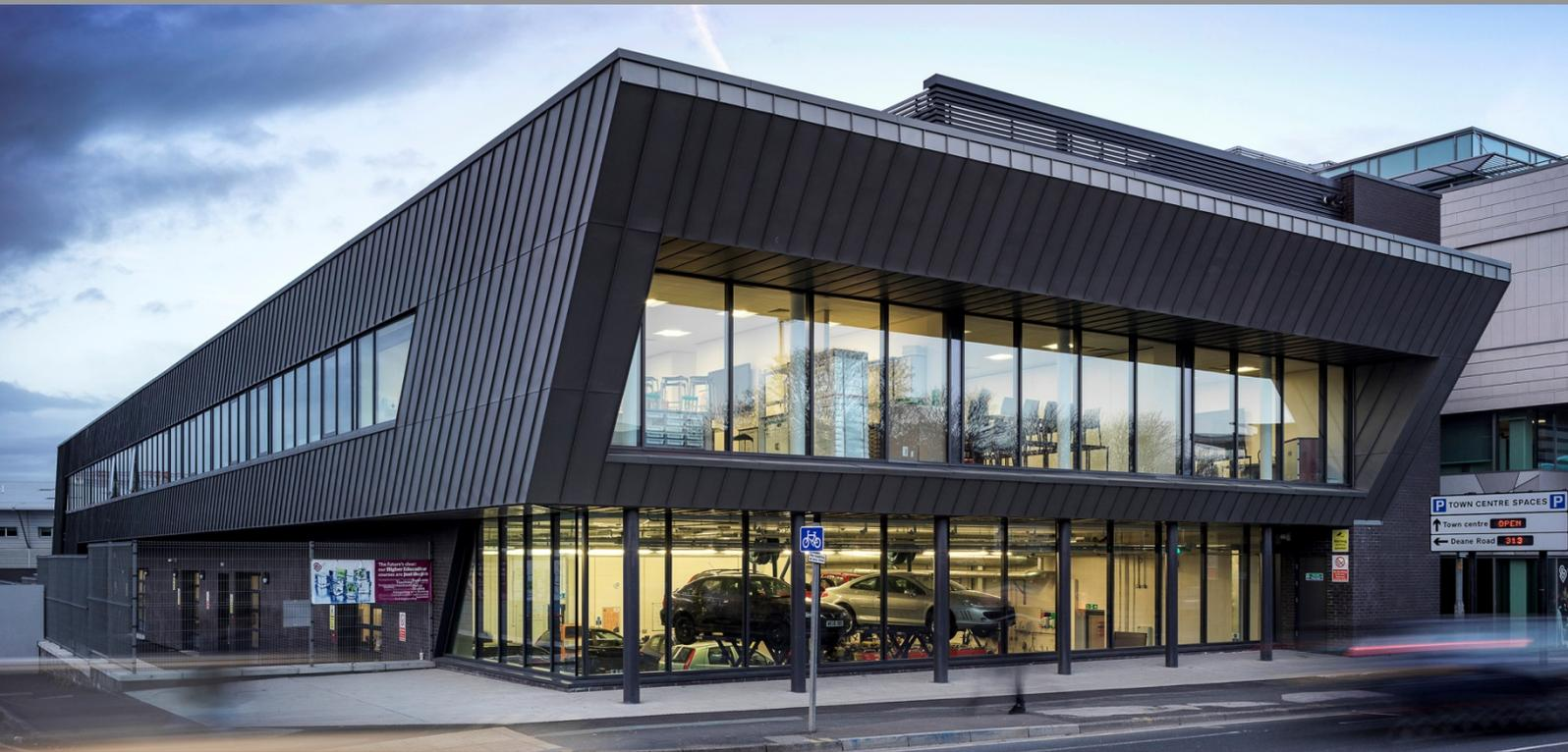
The STEM Centre features a futuristic angled façade which is articulated through the use of angled standing seam zinc cladding completed in NedZink NOVA. Photo: IBI Group
