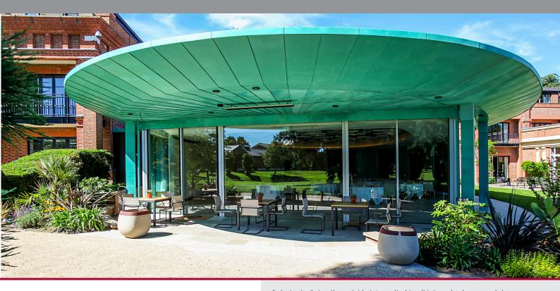
A desire to 'bring the outside in' resulted in all internal columns and door carcasses in the space being covered in the same verdigris sheeting.
