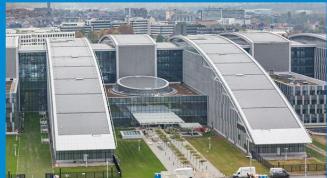
The new NATO headquarters in Brussels has the largest zinc roof in Europe. The roof spans a total surface of no less than 35,000 m<sup>2</sup> of NedZink NOVA Pro-Tec standing seam bays in seemingly unmanageable lengths of 26 metres. A challenging project in many respects.
