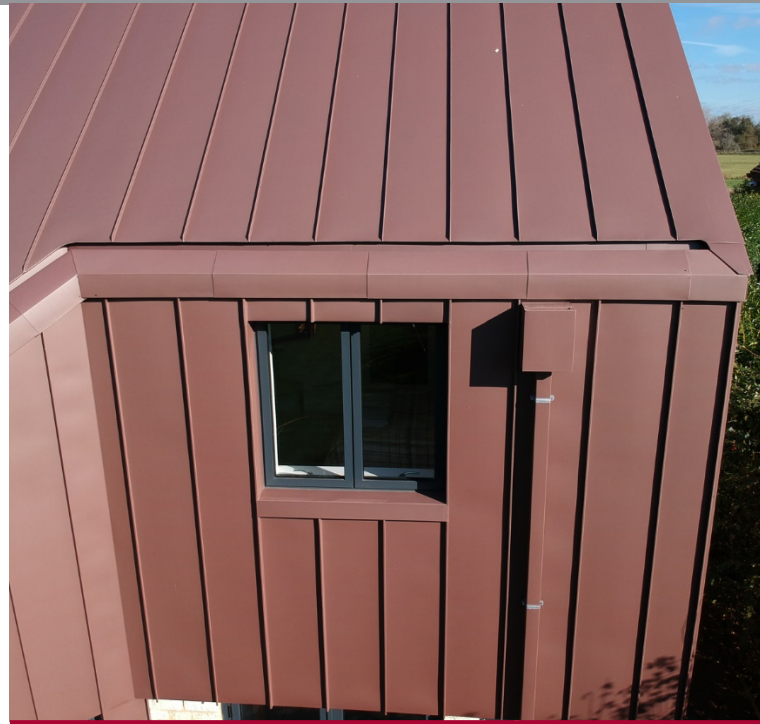
The eaves gutters are pulled back to create a shadow gap along the edge of the roof and free the eaves up from rainwater collection, contributing to the effect of the cladding running over the roof.
